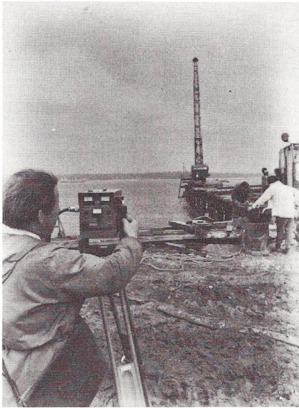
Measuring the centre line for a section of the Humber Bridge.
